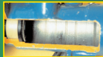
Grooves are worn into the soft metal of the spool valve housing by hardened seals. Metallic debris from such wear accumulates in the fluid causing premature component failure!
